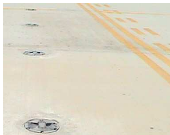
Figure 2: Inset Stop Bars lights and Holding Position Marking
